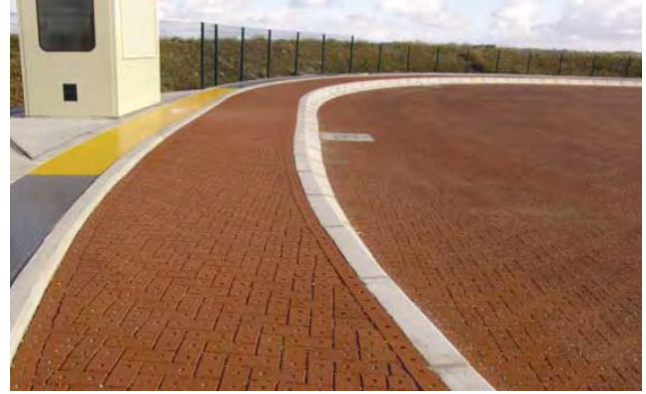
Photo 2 Permeable Clay Pavement
